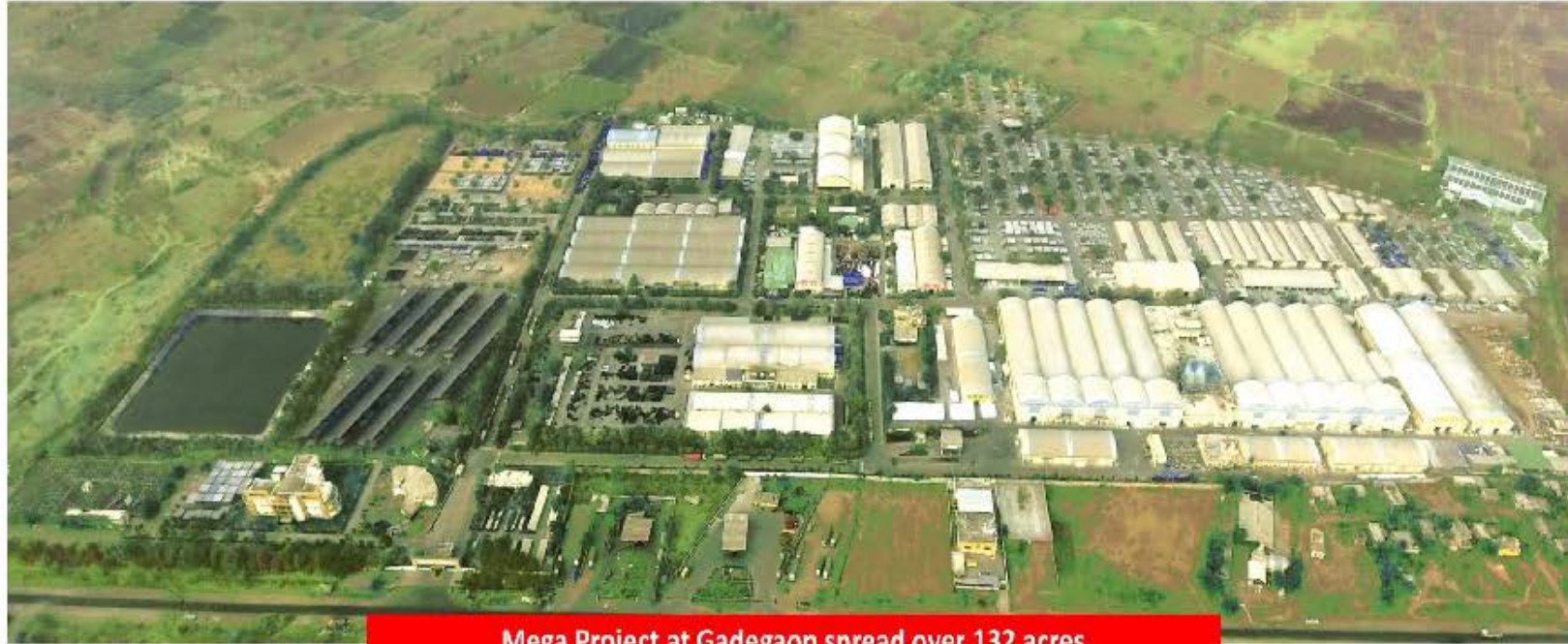
Mega Project at Gadegaon spread over 132 acres
