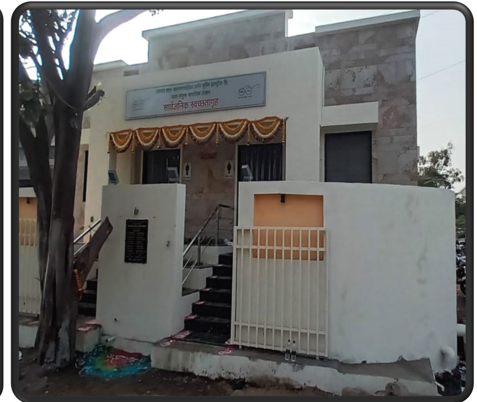
Public Sanitation Facility at Jalgaon (Maharashtra)
