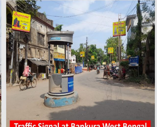
Traffic Signal at Bankura, West Bengal
